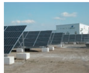
Photovoltaic power plant of RIKEN TECHNOS CORPORATION (within the Gunma Factory site)
